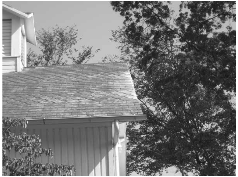
Roof slate on barn roof after repair work.
