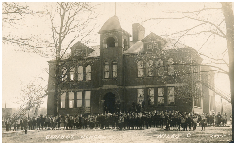
Cedar Street School was built in 1896 and renamed Lincoln School. The building was razed in 1958 and the block of land is now empty.
