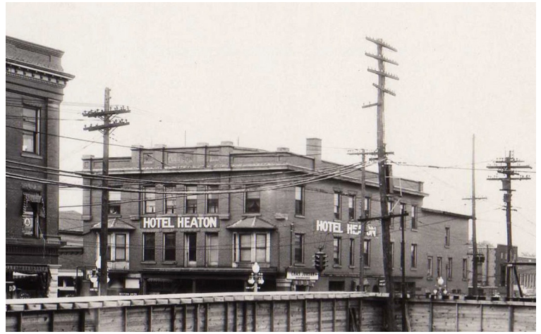
View from the construction site of the Niles Trust Company Bank building with the hotel across Main Street.
