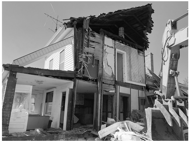
Mason residence shown as it is being demolished. The barrel in the attic would have water pumped up into it to supply water for the shower in the second floor.
