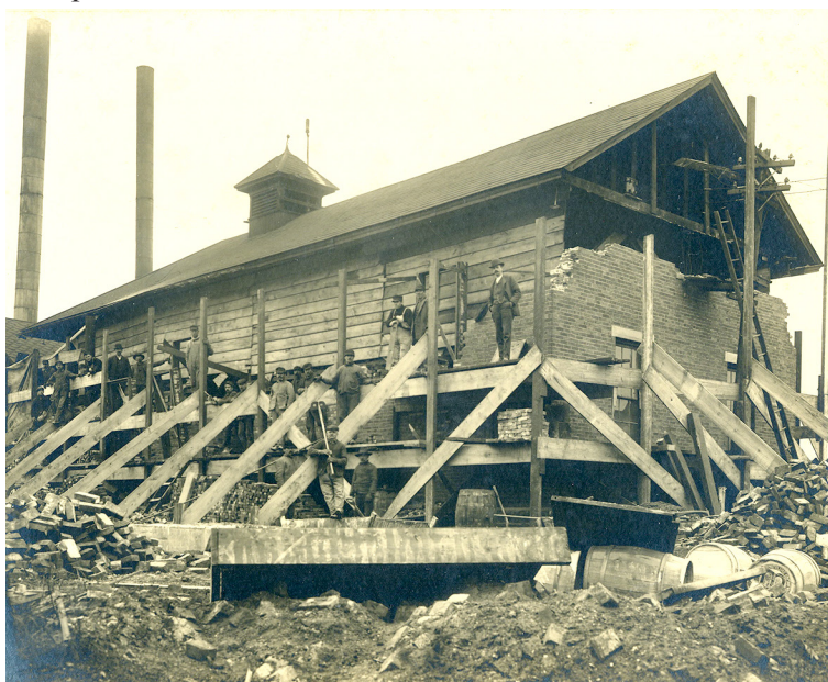
Raising the Niles City Water and Electric plant in 1905.
