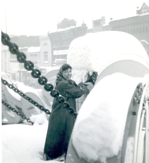
Remember when... Helen Cost Kaniclides worked in the theater building and went out on the Robins Theater marquee sign with a friend to take the pictures of the 1950 Thanksgiving snow storm when over two feet of snow fell.
