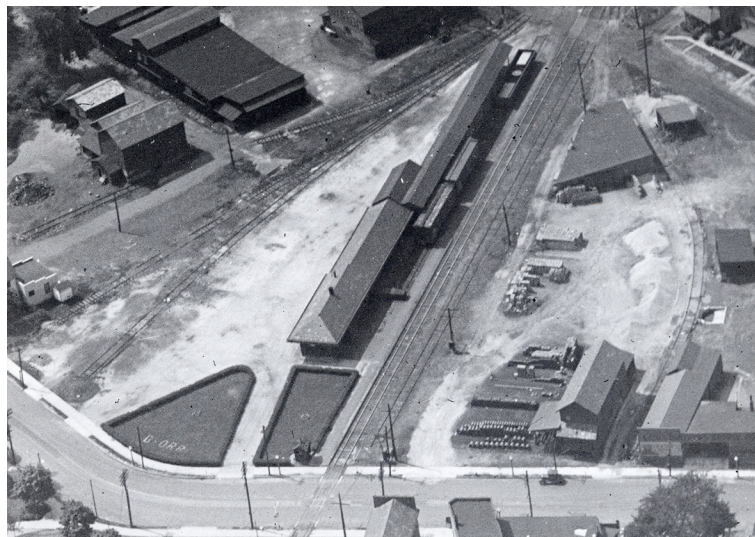
View of B&O railroad yard and Church Street curve before the Grade Elimination Project began in 1953.
