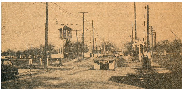
View of North Main Street grade crossing with gates and watch tower guarding the railroad crossover at this location.
