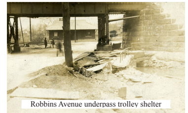
Robbins Avenue underpass trolley shelter
