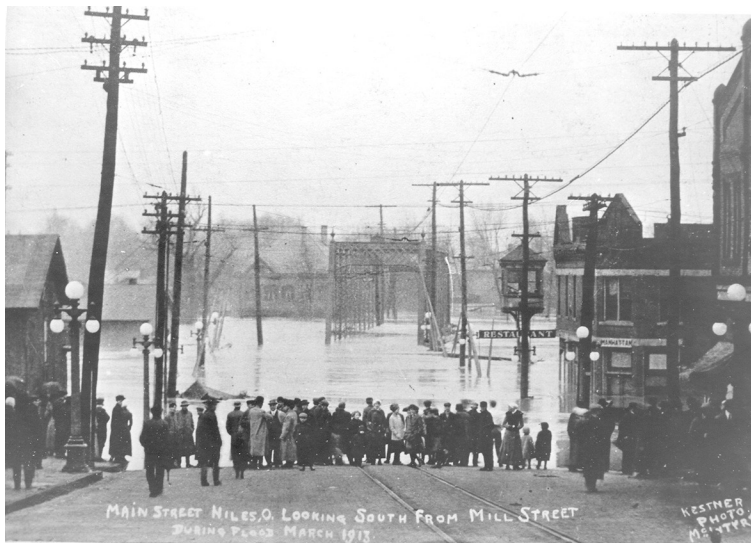
Main Street looking south from Mill Street (State Street) during flood.
