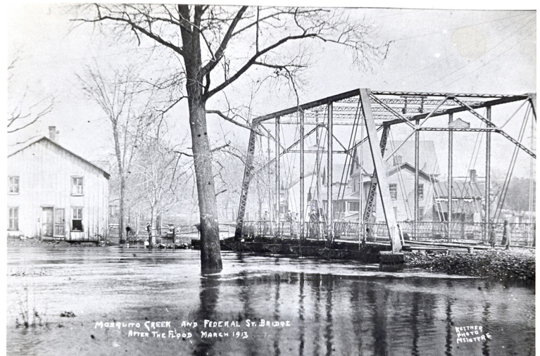
Mosquito Creek bridge over West Federal Street. At the height of the 1913 flood, the water was over the floor of the bridge.
