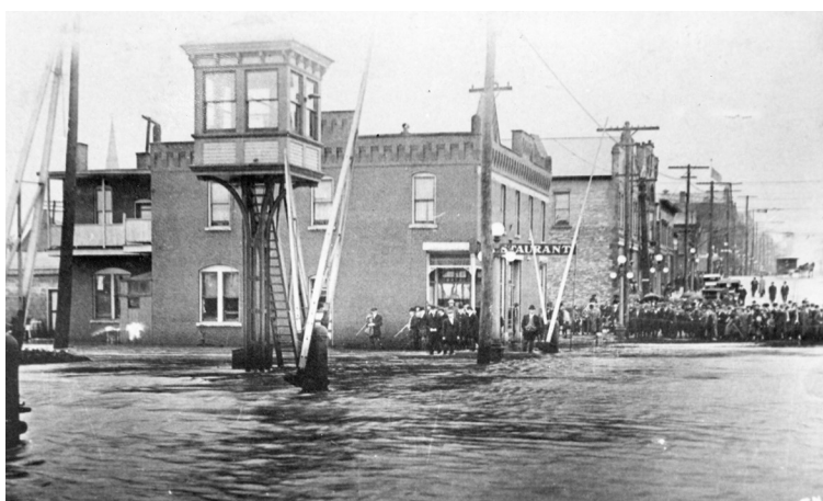
Looking North, the Gilmore Restaurant and Manhattan Hotel on South Main Street and Water Street during the 1913 flood.
