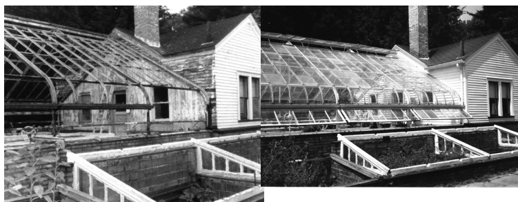
Greenhouse during refurbishing and after the work had been completed.
