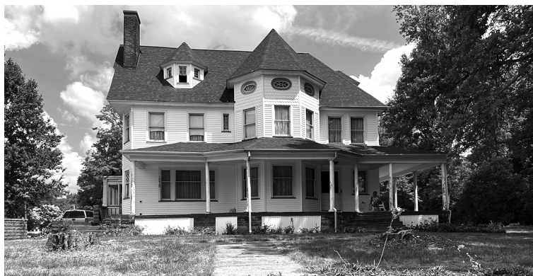
Harry Stevens residence undergoing renovations in July 2022.
