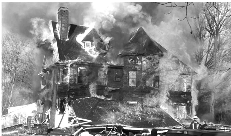
The Harry Stevens Home, engulfed in flames, was totally destroyed.
