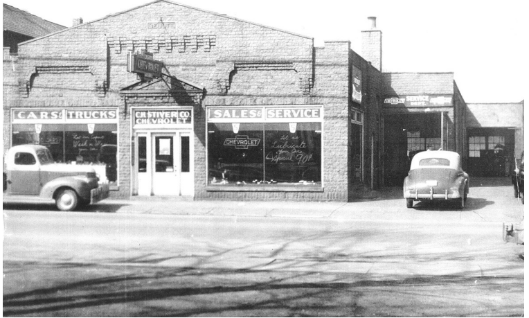
The DeJute Building at 236 North Main Street was built in 1928. A Desoto-Plymouth dealership was then located here. Later, C.H. Stiver sold Chevrolets at this location, then moved across the street.
