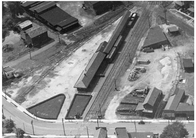
Aerial view of the B&O railroad yards showing the path of East Church Street before the overpasses were built in 1953. Also note that East State Street did not continue through to Robbins Avenue at this time.
