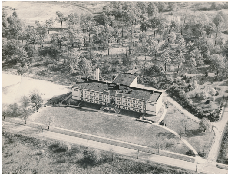
Aerial View Of The East Side Junior High School Known As Washington.
