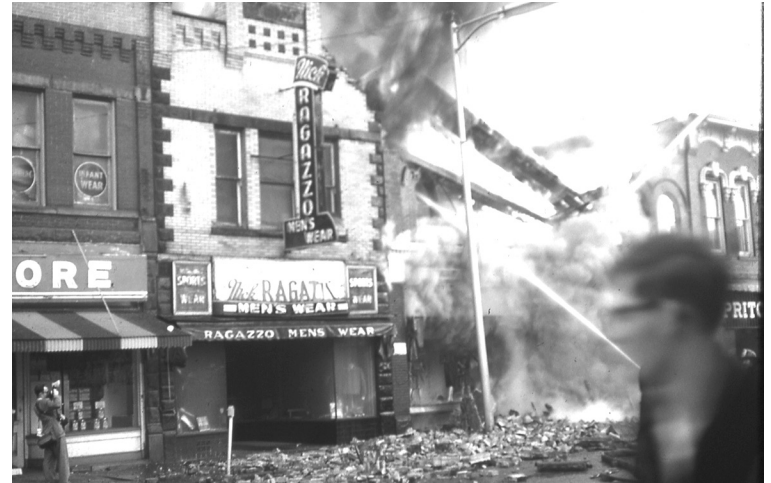
Above: Hoffman's Department Store building collapses from fire.
