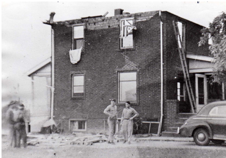
Home of Dominic Mauro on North Road was badly damaged. The roof was ripped completely off and the interior heavily damaged.
