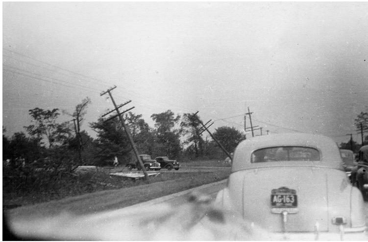
The path of destruction left by the 1947 tornado and even the funnel cloud (upper right corner) is visible in this photograph.
