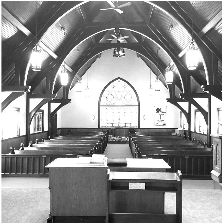
Interior view of St. Luke's Episcopal church looking from the pulpit toward the main stained glass windows that face Robbins Avenue. The roof is supported by arched wooden beams anchored to the walls.
