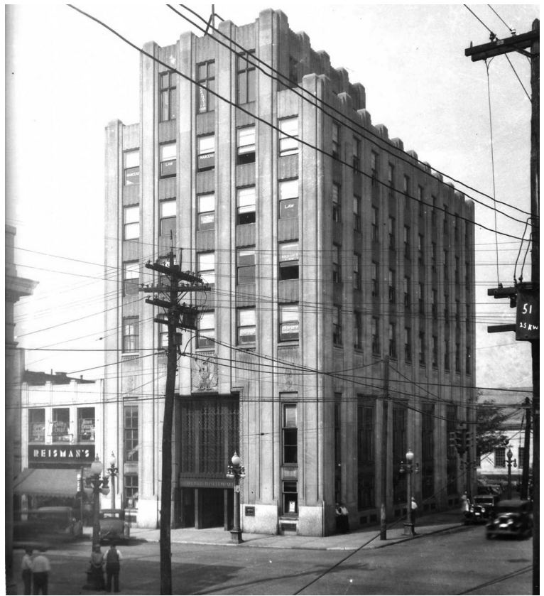
Between the Holeyton building (1887), occupied by Kreiger's Pool Hall, and the bank, a new building was erected and occupied by Reisman's.
