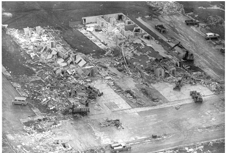
Aerial view of the May 31, 1985 tornado damage to the buildings at Route 422 and Niles-Vienna Road.
